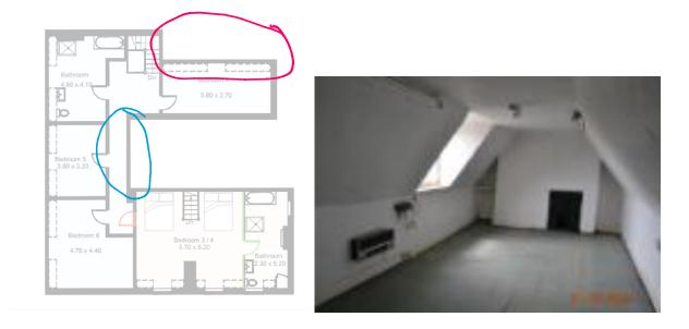
Highlighted in red The bedroom wall is not stepped in as shown, the chimney breast is missing and the dormer appears to be off centre rather than the position shown on the drawing.
